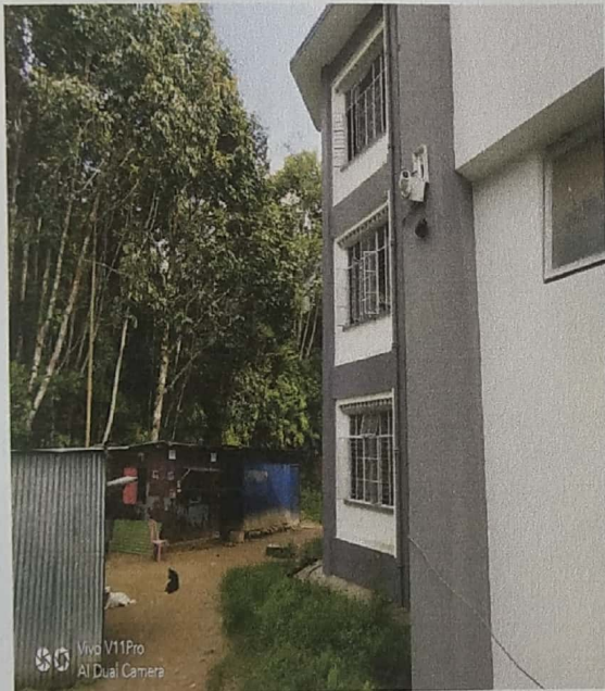
Photo 2: CCTV installation in the college premises which is monitored 24/7.
